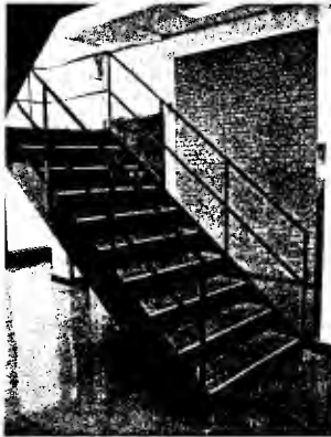
Figure 32. CRB connection wing staircase.
